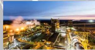
Western Australia Synthetic rutile kiln Cataby project
