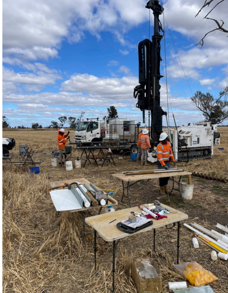
Geotechnical drilling taking place on the Wimmera Project site
