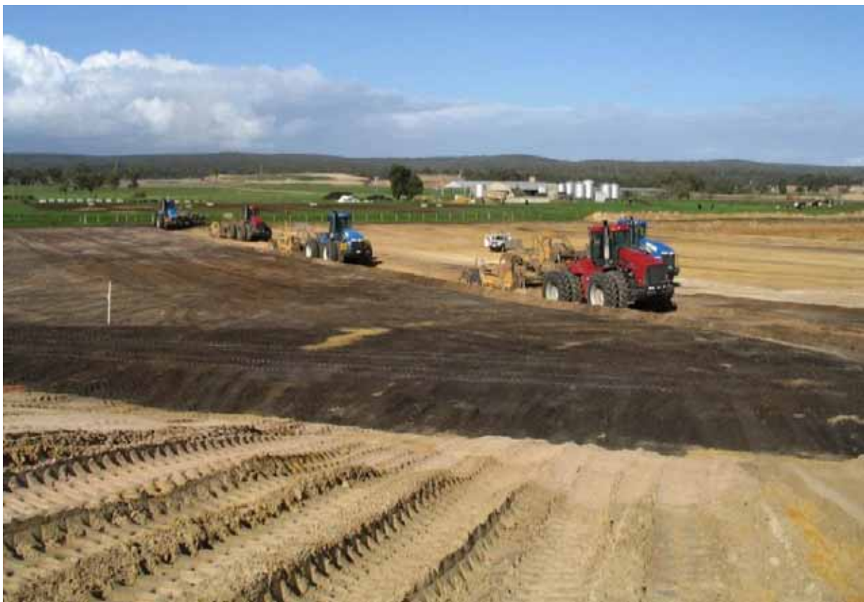
Plate 14: Soil replacement operation at Echo mine
