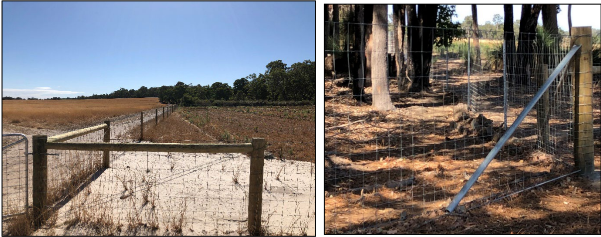
Plate 4: Internal Stock Fence (left) and 1.5m Boundary Fence (right)
