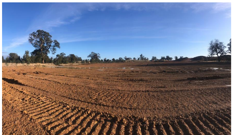
Pit 21 backfilled to design surface, April 2022
