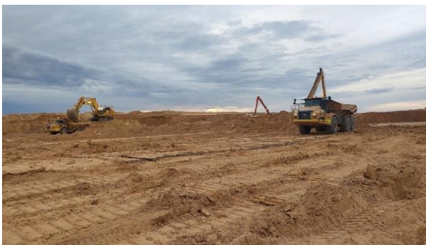
Earthworks commence at the Eneabba site
