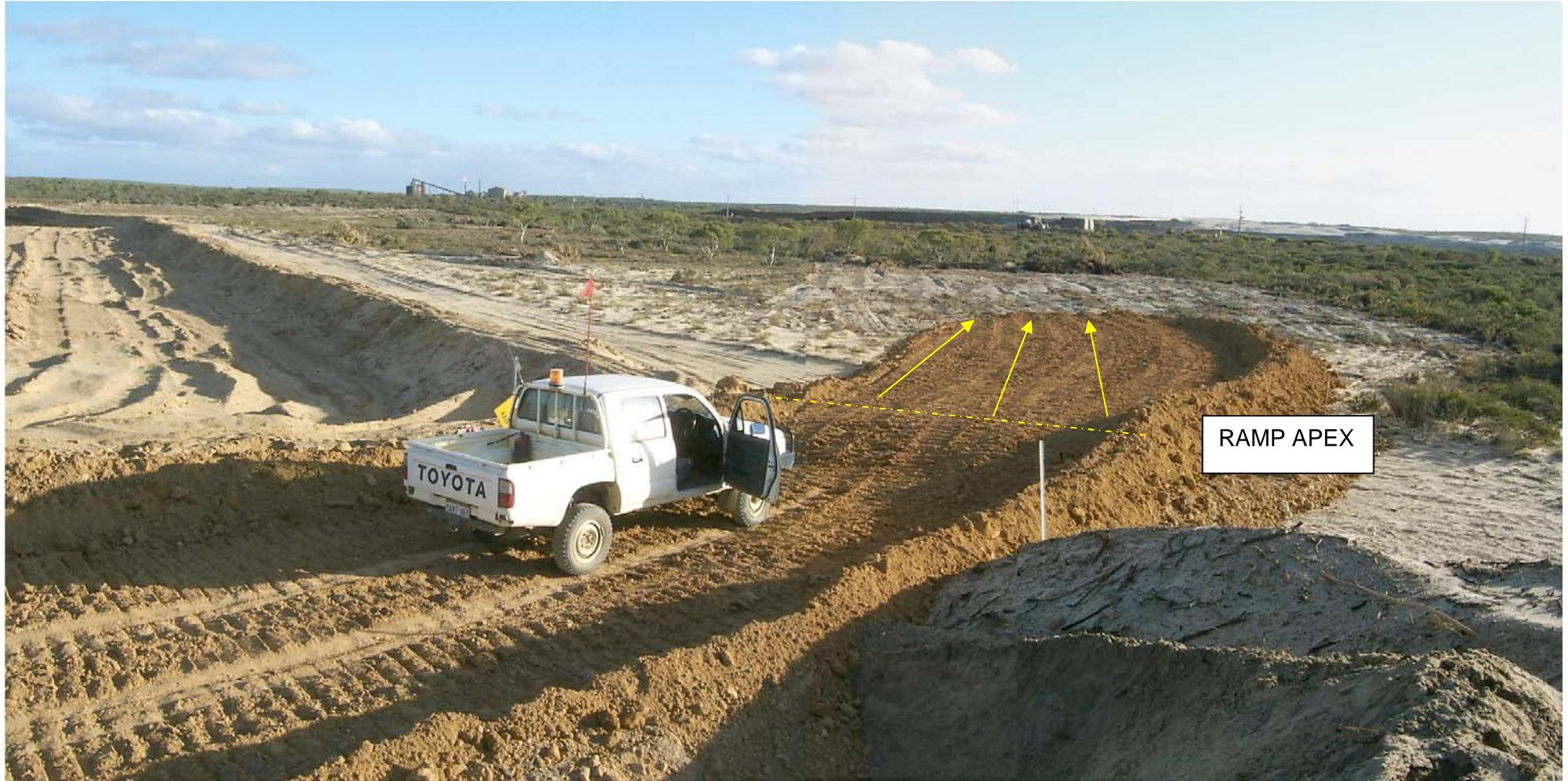
Hygiene ramp constructed with oversize material. Ramp section steps up immediately in front of LV with wash water returning to dieback infested area (vegetation in background)
