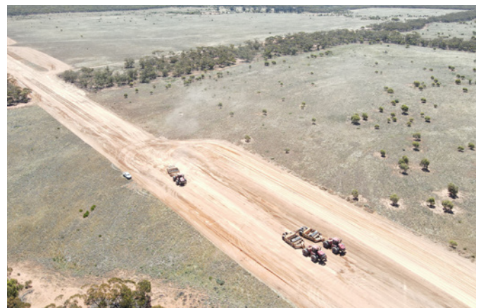
Construction of the haul road to the Balranald site
